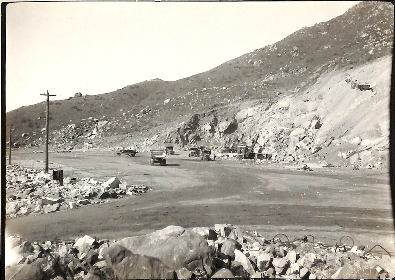
12-3-32 C. S. D. El Capitan Dam. Looking Westerly Along Quarry Floor.
