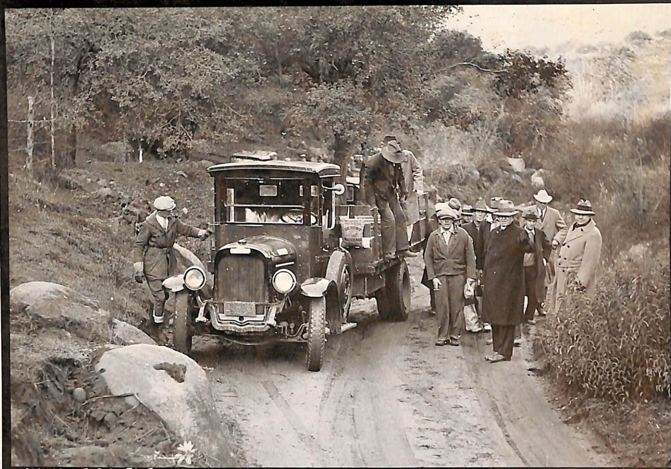
12-23-31. C.S.D. El Capitan Dam. Inauguration of Work. First Laborers Arriving. E.C-4.
