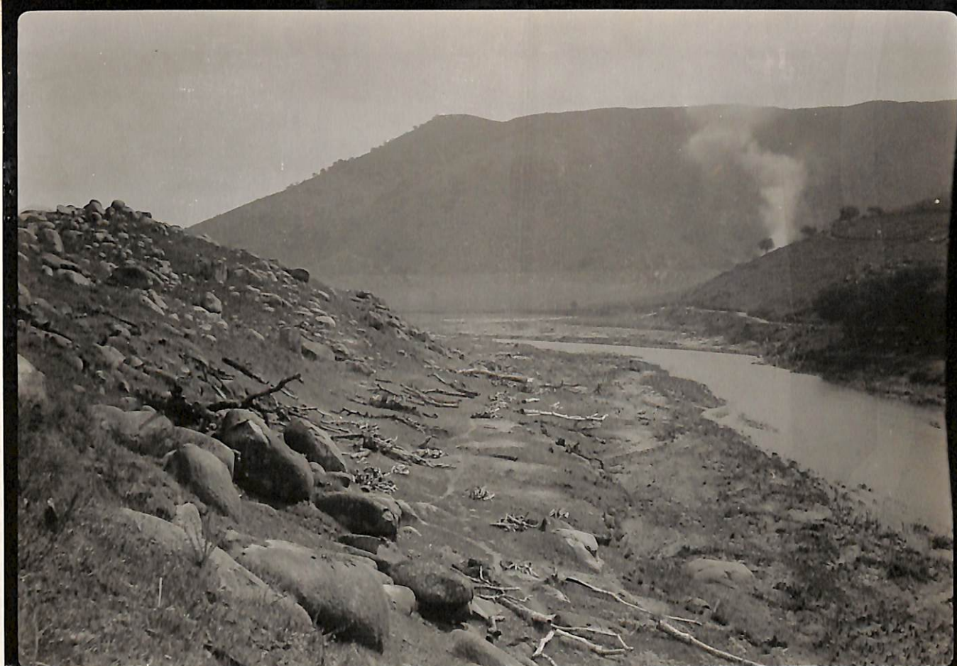
3-14-32. C.S.D. El Capitan Dam. Looking Upstream from Vicinity Damsite No. 1. EC-42.
