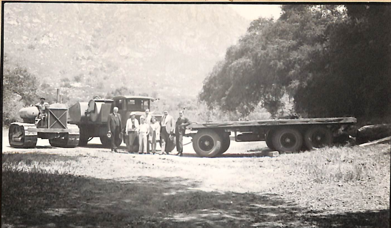
4-24-32. C.S.D. El Capitan Dam. Contractor's Outfit Arriving.
