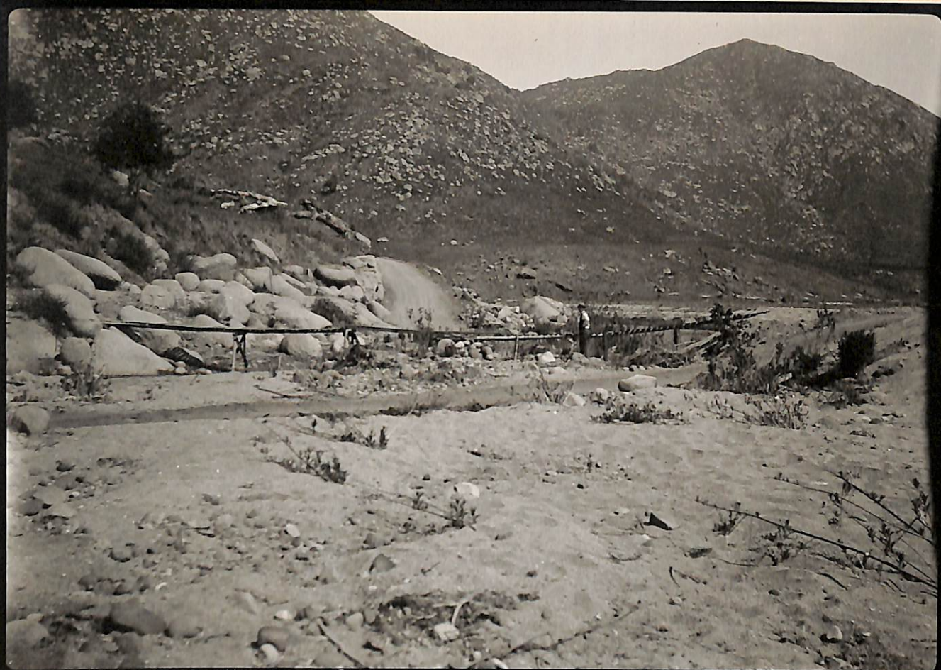
4-6-32. C.S.D. El Capitan Dam. Chocolate Creek Foot Bridge Looking North.
