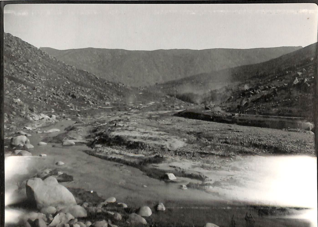
1-25-32. C.S.D. El Capitan Damsite. Looking Upstream.
