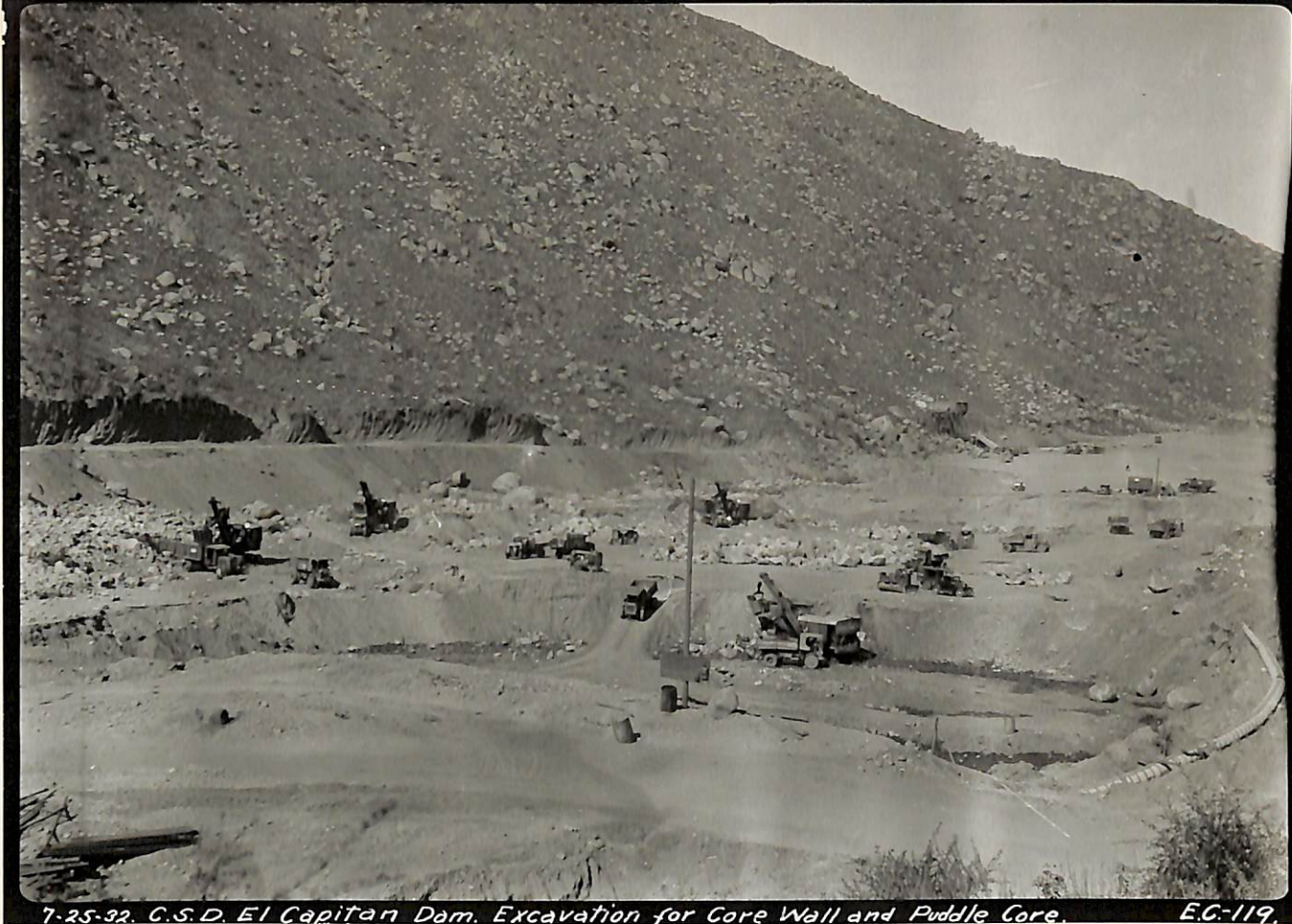
7-25-32. C.S.D. El Capitan Dam. Excavation for Core Wall and Puddle Core.
