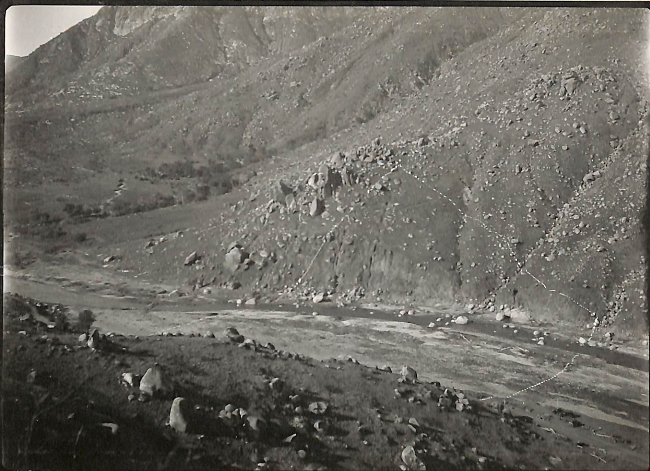
1-22-32. C.S.D. El Capitan Dam site. Right or North Abutment.
