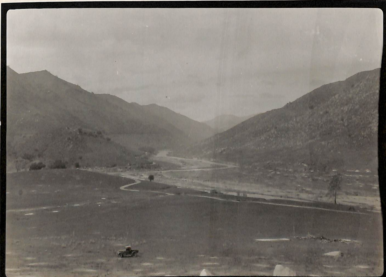
3-14-32. C.S.D. El Capitan Dam. Looking Downstream Material Area "A"
