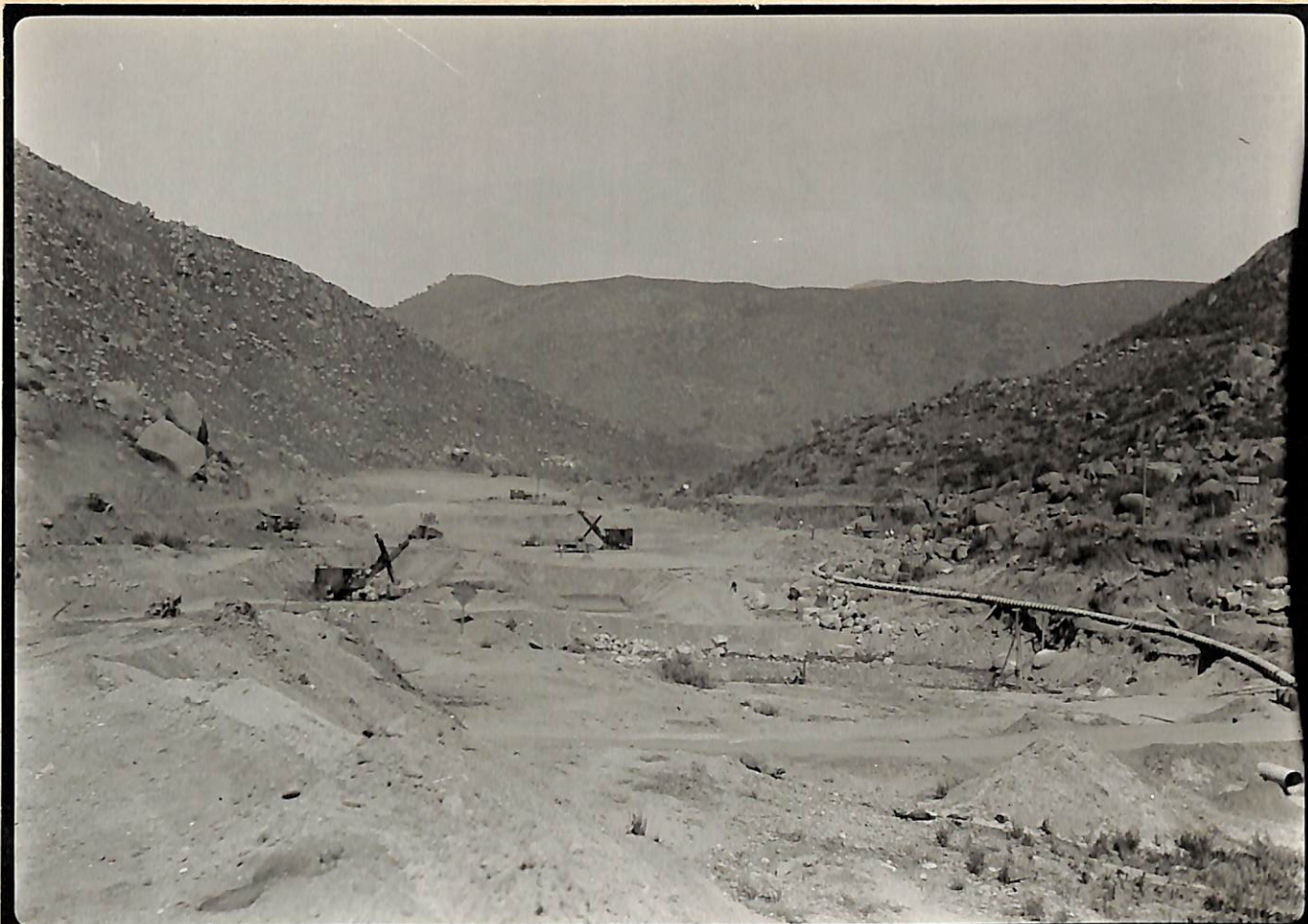
7-11-32 C.S.D. El Capitan Dam site Looking Upstream.
