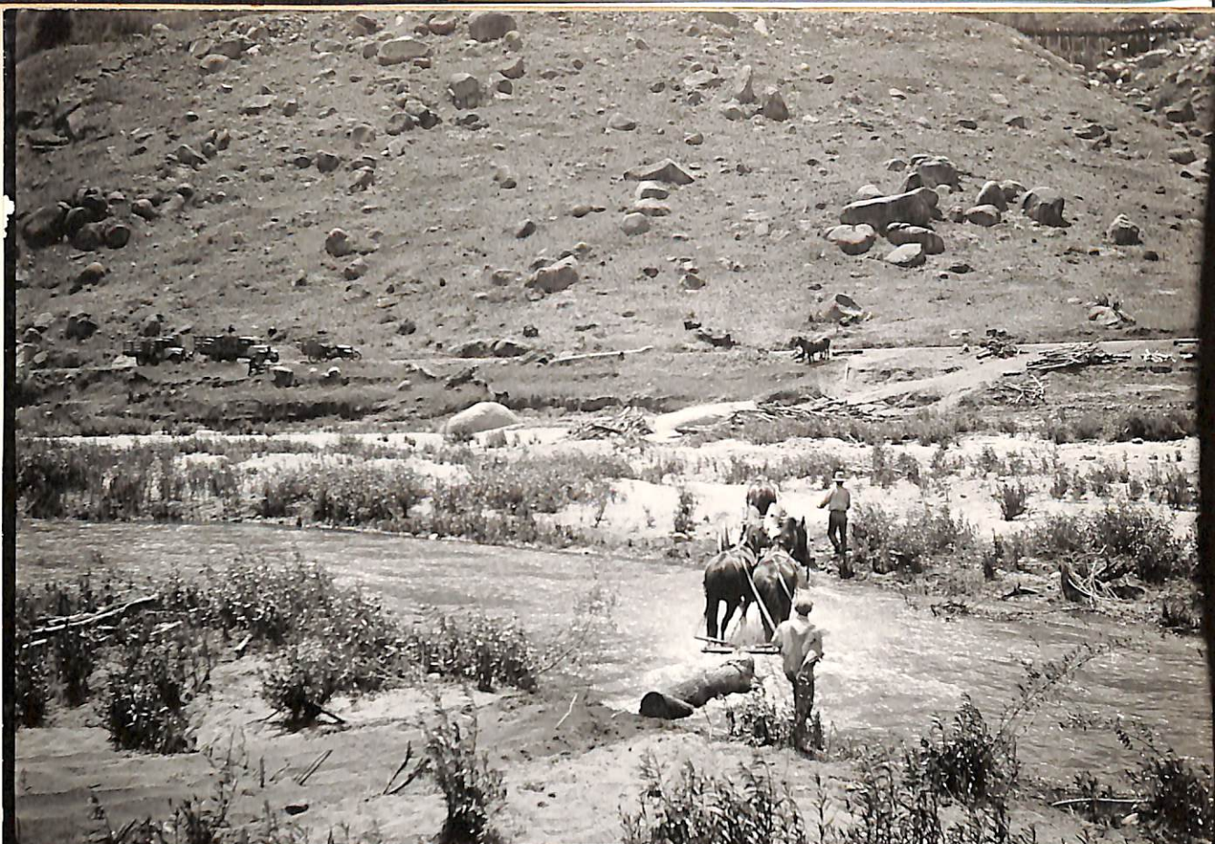
4-15-32. C.S. D. El Capitan Dam. Removal of Wood by The Public.
