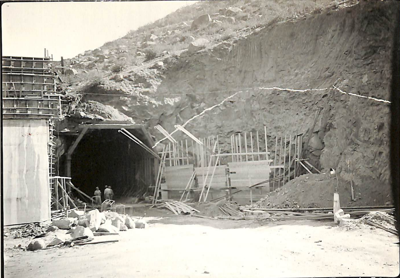
10-28-32. C.S.D. El Capitan Dam. Discharge Portal of Diversion Tunnel. E.C.198
