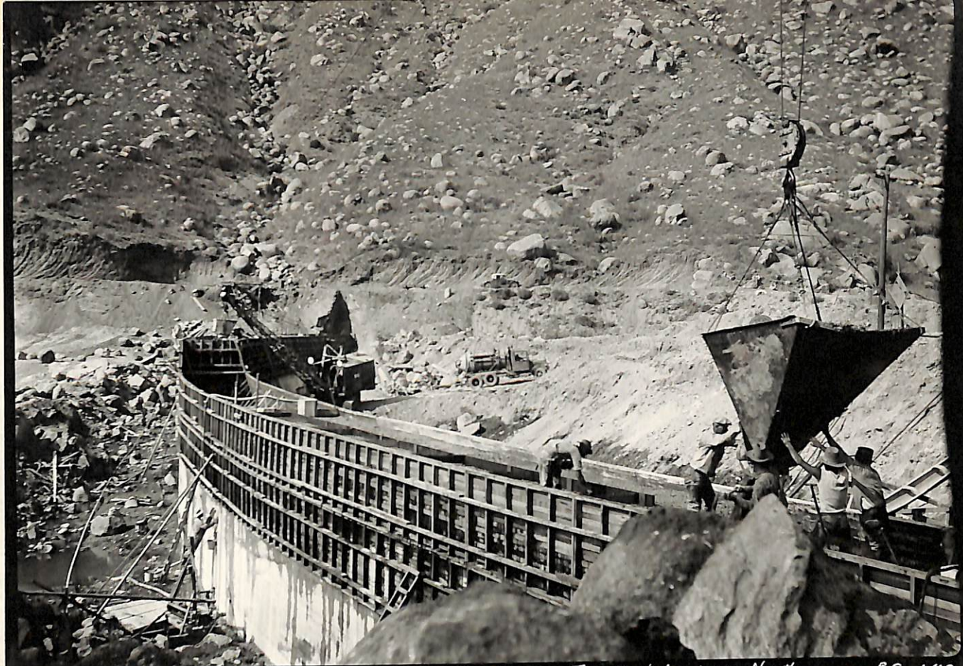
8-29-37 C.S.D. El Capitan Dam. Pouring Upstream Toe Wall - Looking North
