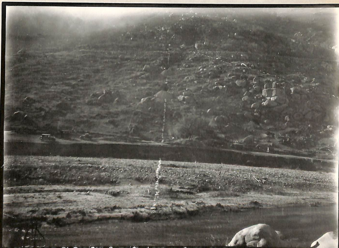
1-29-32. C.S.D. El Capitan Dam site. Left or South Abutment.
