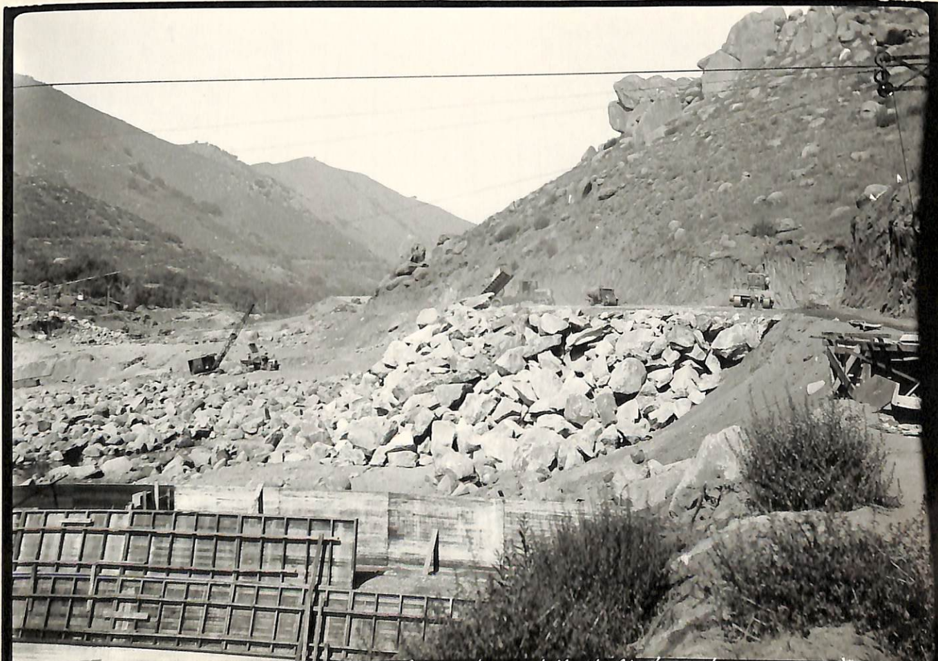
9-1-37 C.S.D. El Capitan Dam - Rock Embankment North Abutment
