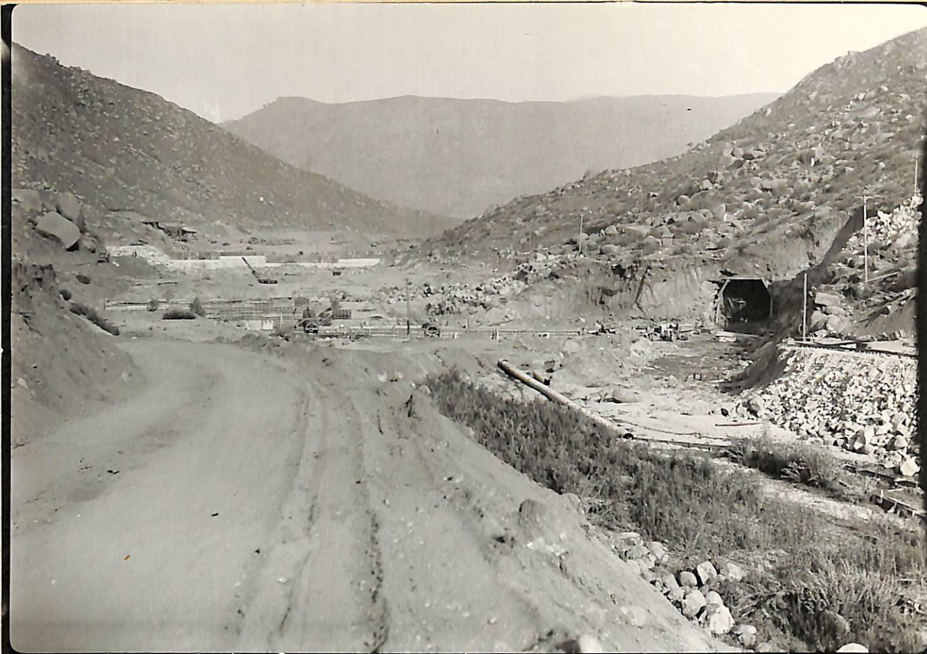
9-8-32 C.S.D. El Capitan Dam - Looking Upstream From Downstream Spoilbank. EC151
