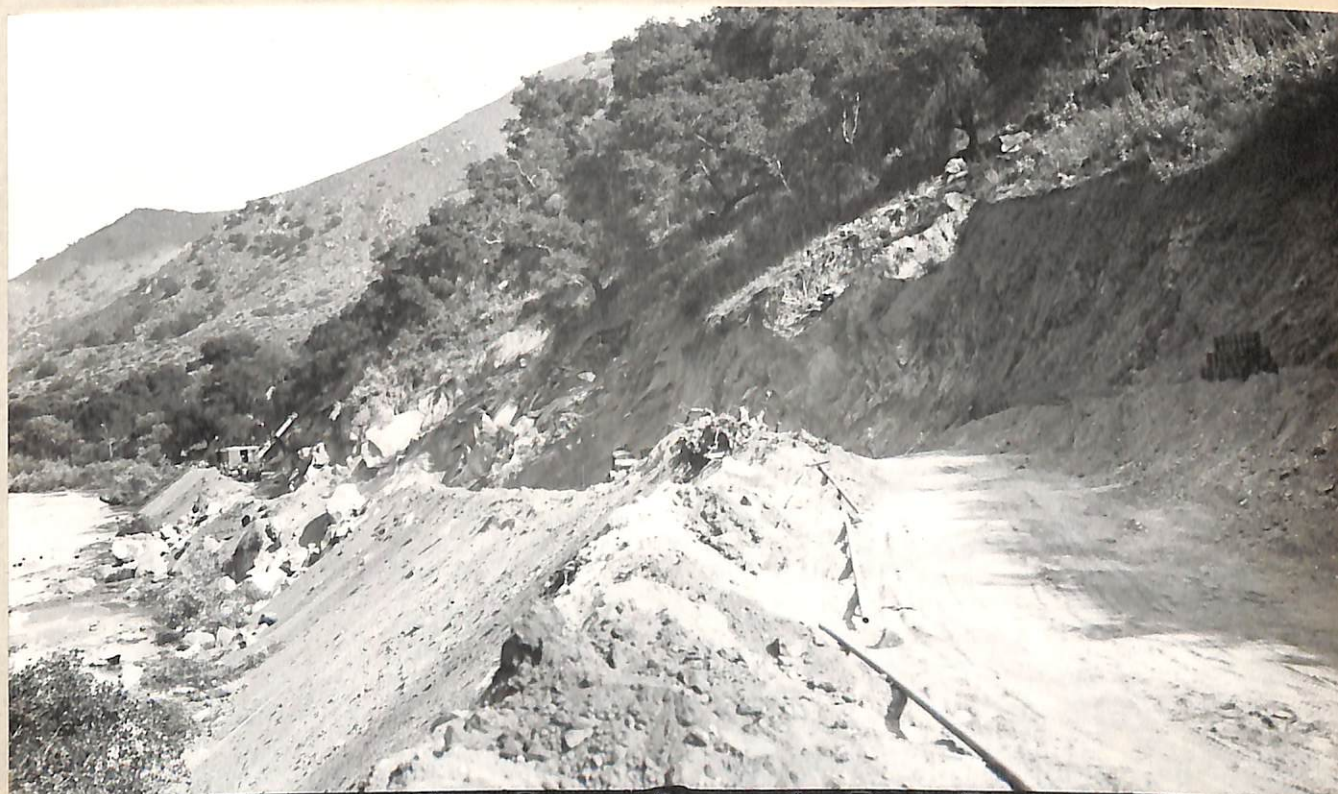
5-3-32. C.S.D. El Capitan Dam - El Monte Park Road, P.L. Mile 1 1/2.
