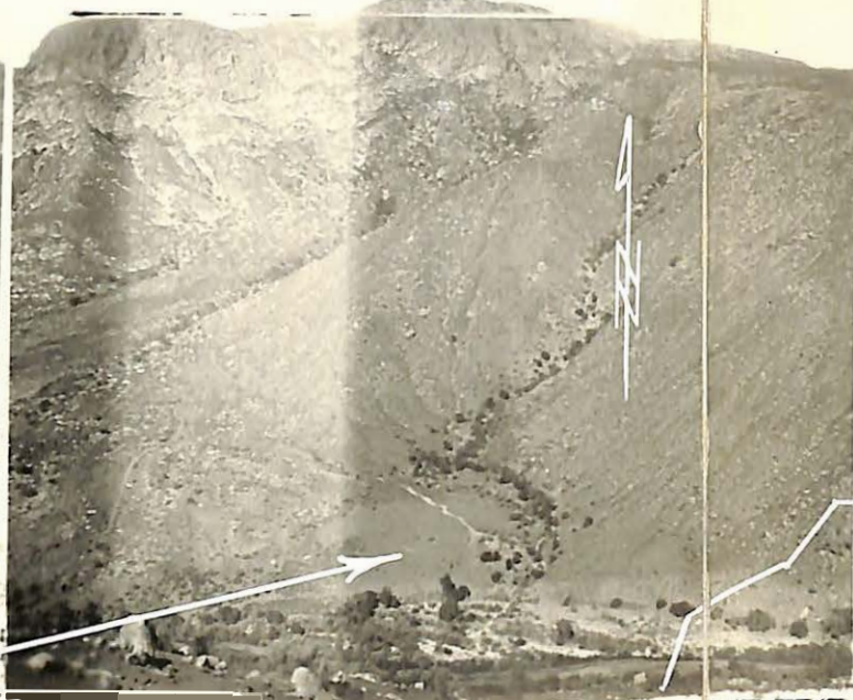
Hydraulic Fill Site "C"
