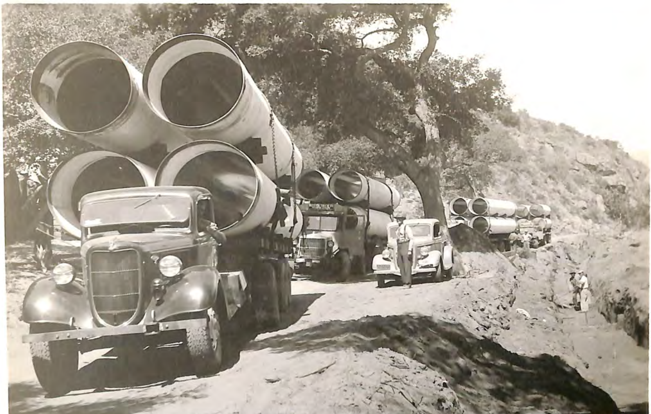
6-29-36, C.S.D. El Capitan Pipe Line - Delivering pipe to job.
