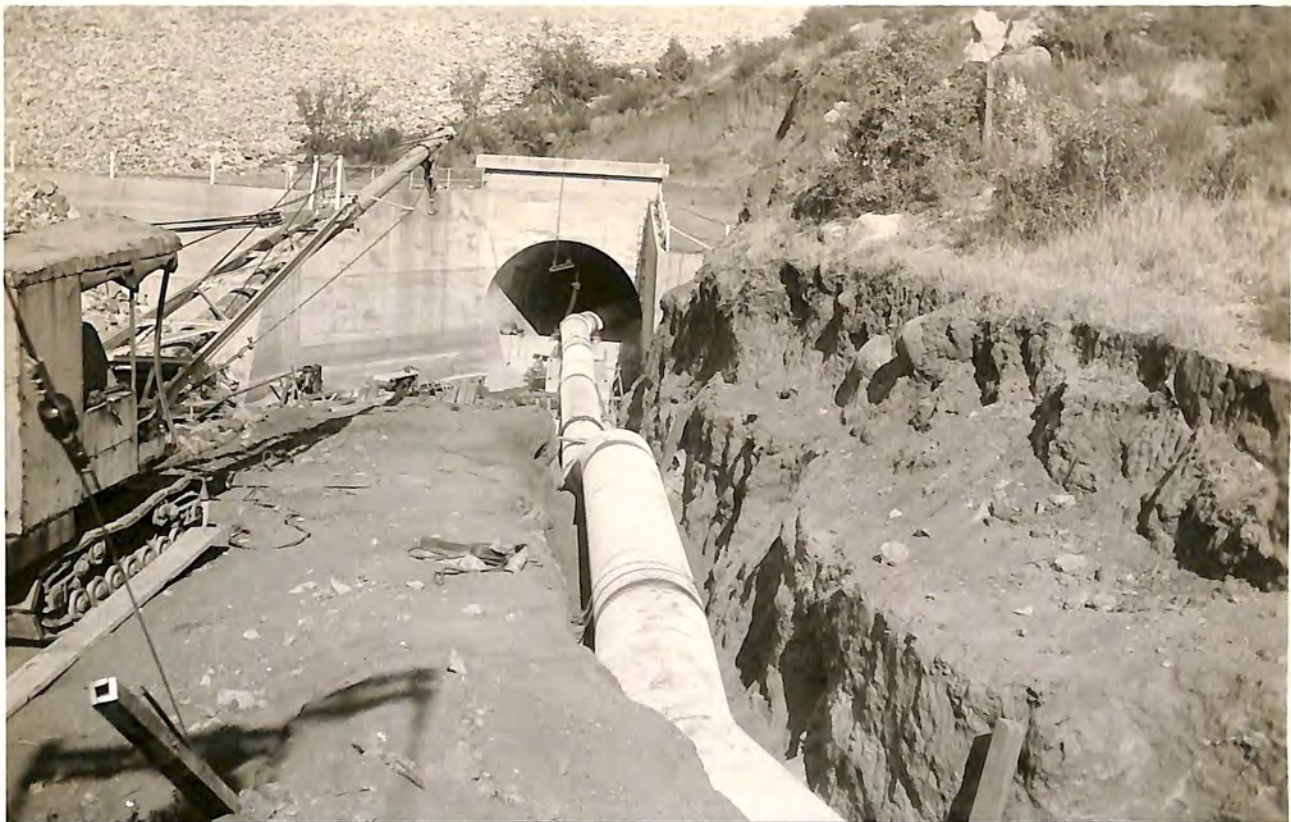
6-29-36-C.S.D. El Capitan Pipe Line - Looking upstream from 13+00. EC-942
