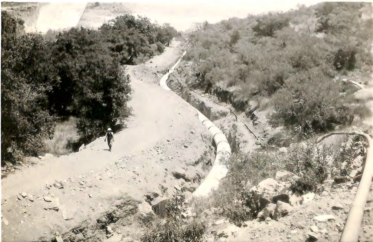
7-13-36 C.S.D. El Capitan Pipe Line. Upstream from 29+25 EC 946
