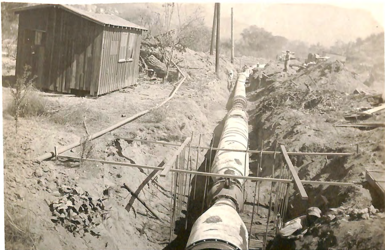
9-28-36, CSD, El Capitan Pipe Line - Downstream from Sta. 311+56
